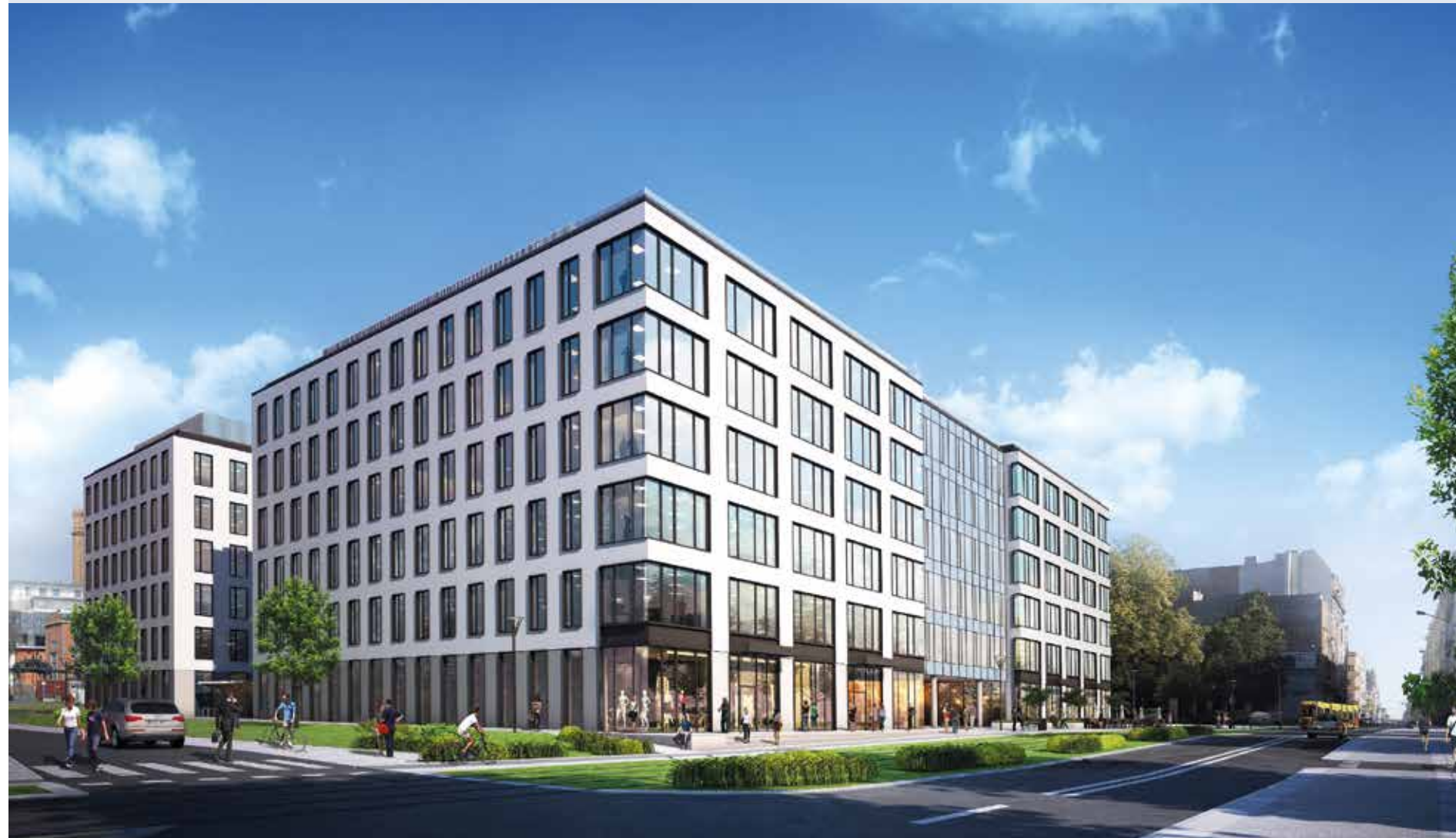
"MBANK STOP" OFFICE AND CONFERENCE CENTER
