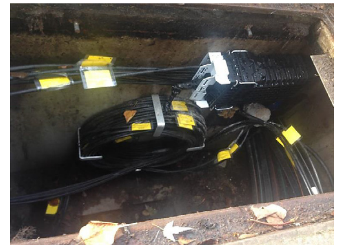
Fiber optic access network
